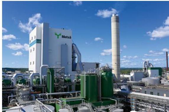
Figure 2. Boiler building, Metsä Group, Äänekoski, Finland. White and light blue walls of the large building are made using horizontal sandwich panels from column to column ( photo: https://www.ruukki.com/fin/b2b/referenssit/reference-details/mets%C3%A4-group-biotuotetehdas-%C3%A4%C3%A4nekoski )
