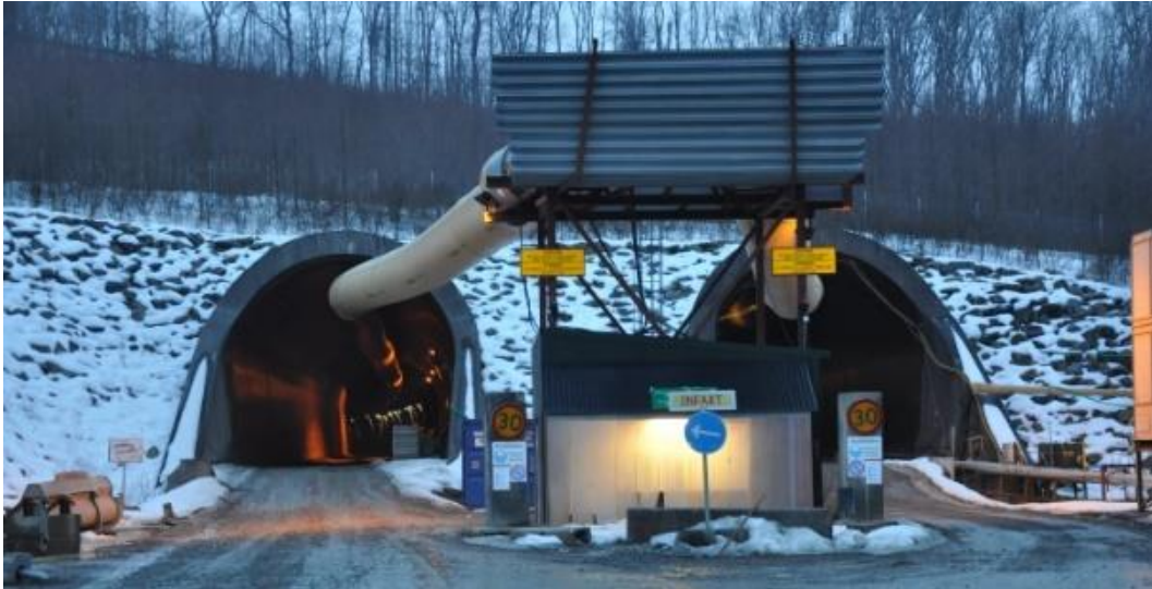
Figure 1. The Hallandsås tunnel during construction.
